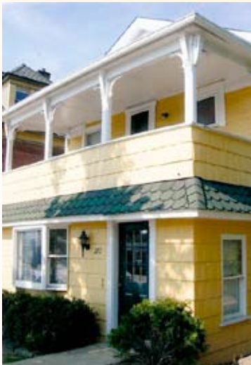
277 South Court Street. This small Greek Revival home (style popular in the U.S. from 1820-1850) was given some Victorian embellishments in 1880 in the form of a second story porch and Victorian gingerbread trim.
